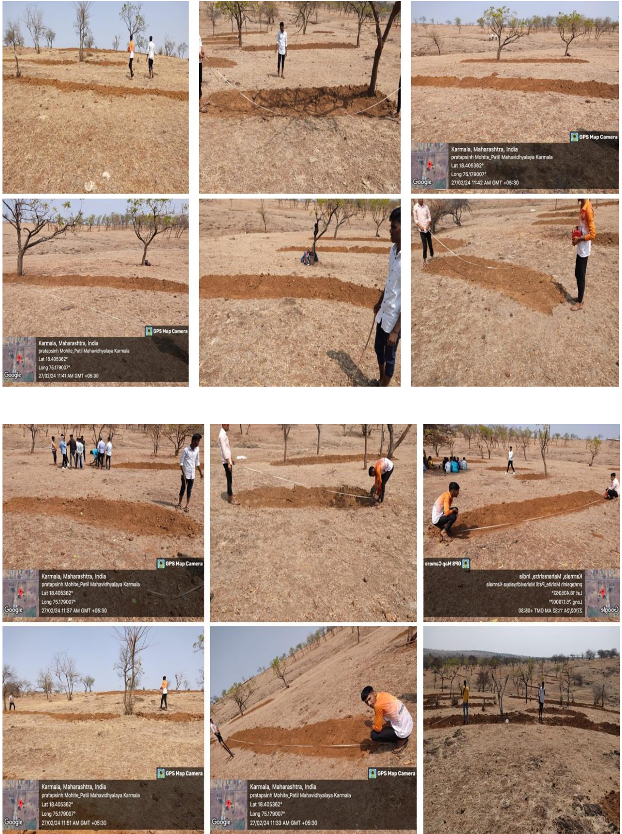
Water Conservation through Construction of Continuous Contour Trenches (CCT) in Roshwade
